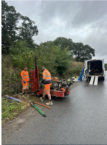
Window sampling rig positioned at the exploratory location
