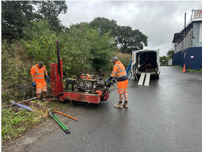
Window sampling operations at The Old Orchard
