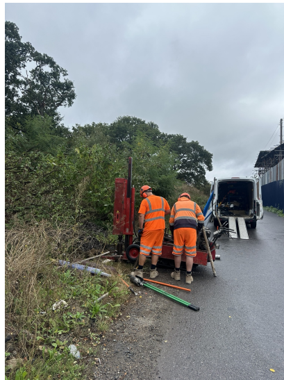
Site investigation rig and sample trays during the works
